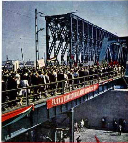
THE MAIN RAILWAY BRIDGE over the Danube at Budapest is opened, and workers who helped in its rebuilding walk across behind the first train. Banner on bridge reads: "Long Live the Soviet Union, Strongest Guardian of Peace."
