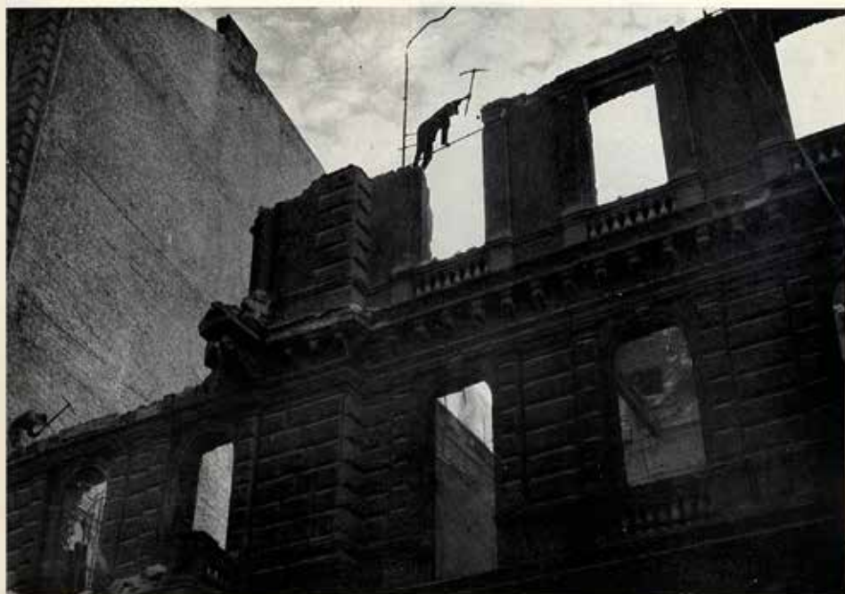
BUDAPEST IS REBUILDING slowly, and mostly by hand. On top of the old Ritz Hotel tiny figures attack the walls with picks.
